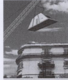
Penthouse construction in Buenos Aires
